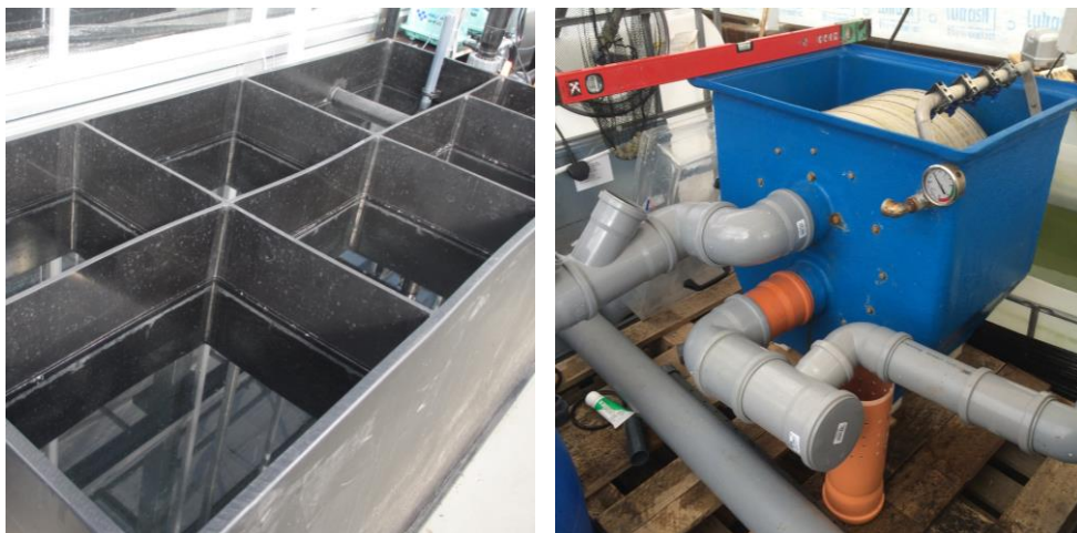
Figure 3.2 Sedimentation tank (left) and drum filter (right)
