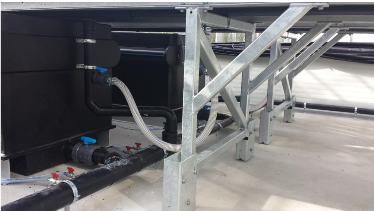
Picture 1. IGFF Legging of mobile plant tables, and supplied with flexible soft piping that leads the water from the plant tables back to the sump tank during ‘flood and ebb’ on the tables for feeding the plants.
