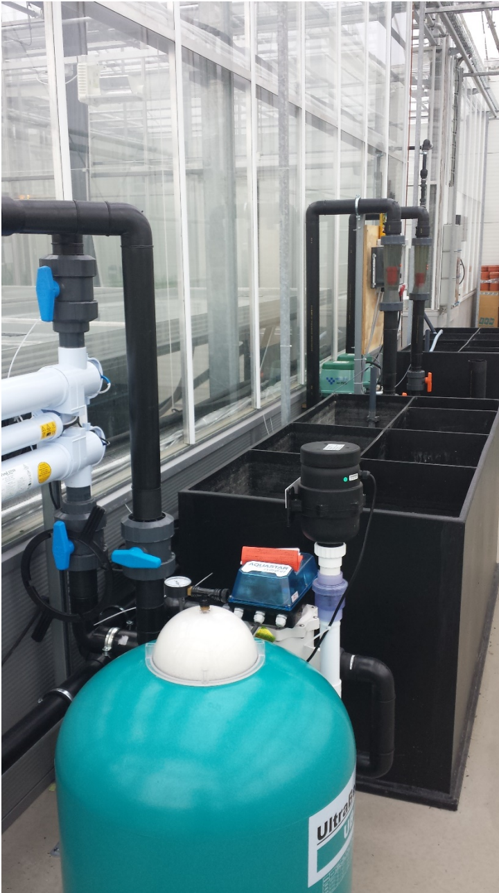
Figure 3. Bio-filter, UV-lighting, sedimentation tanks and airblower.
