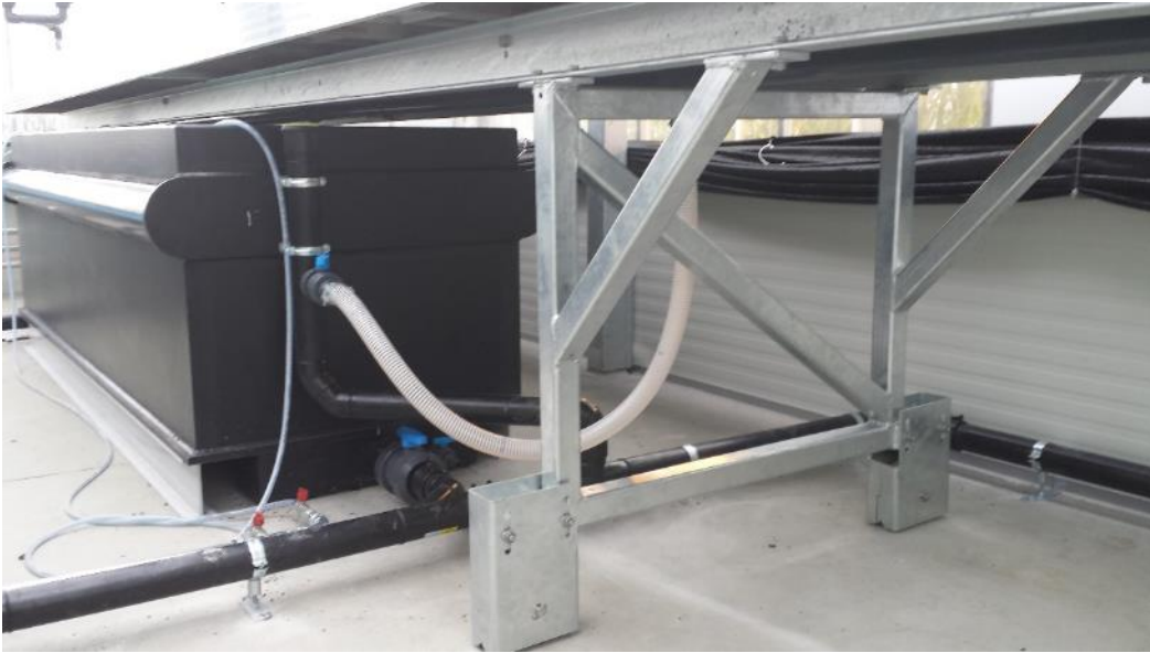
Figure 1. Special legs invented to secure mobility of the plant tables above the fish tanks, and so secure high savings on space and fixed cost.
