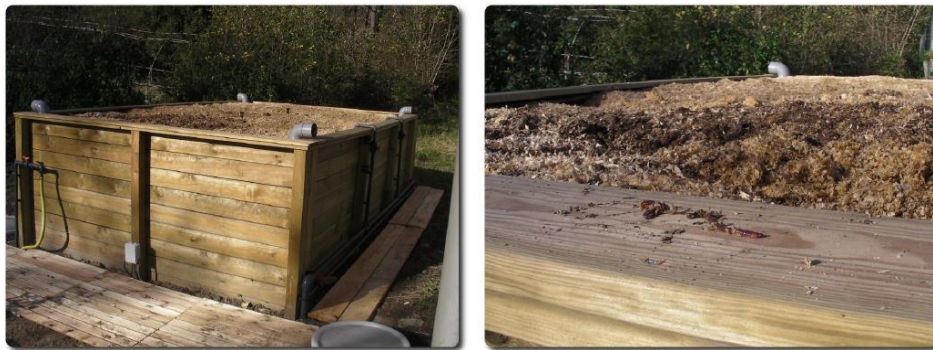
Vermiculture: biological sewage treatment plant at BREEN demonstration plant
