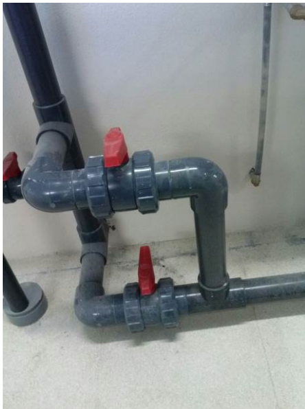
Figure 7. Stopcock system to release sedimentation.
