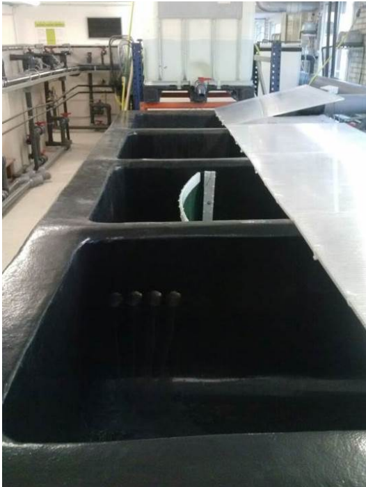
Figure 3. A four compartment settling tank forms the filter system at Breen together with three sand filters.
