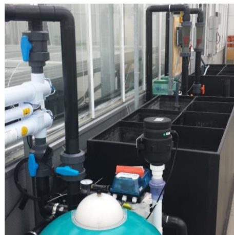
Figure 2.7 Bio-filter, UV-lighting, sedimentation tanks and airblower
